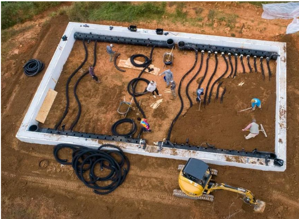
Figure 1: GAHT Construction Image
